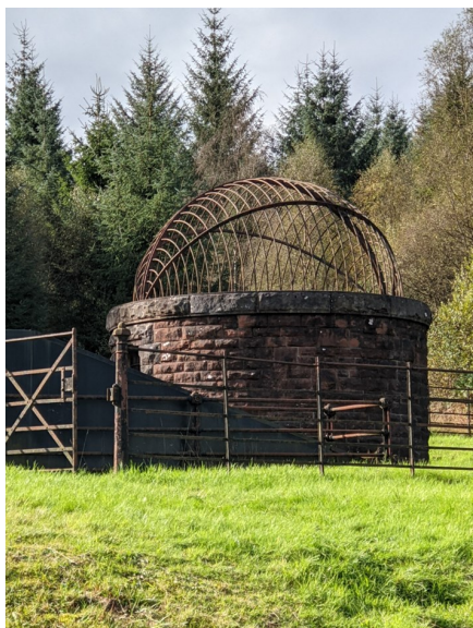
Air vent—part of the Water Supply from Loch Katrine
